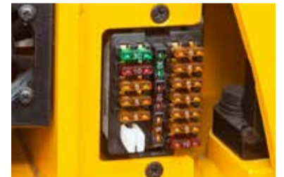
Concentrated fuse box
